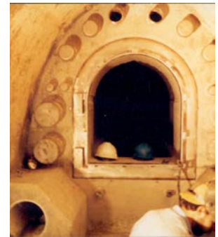
“Chicago Tunnel Project (1992) Flood”
